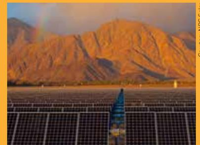
The NRG Solar Borrego I Project consists of 102,000 photovoltaic panels, each one measuring roughly 3 feet by 6 feet, installed on 308 acres owned by NRG Solar in the Borrego Valley.
