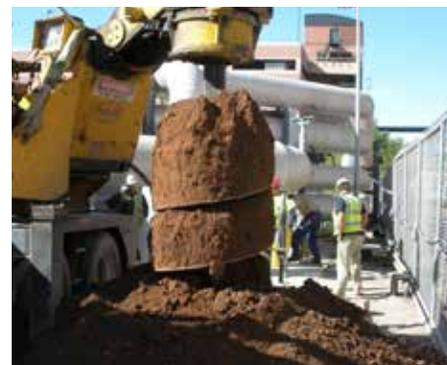
Crews drilled 12 new holes and used four existing ones for the caissons to support NRG Phoenix's new cooling towers. The caissons—concrete columns drilled and cast into the ground as foundation supports—are each 15-feet high and 36 inches in diameter.
