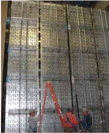
Taken from the ice tank floor, this image provides perspective on the size of the new coils.
